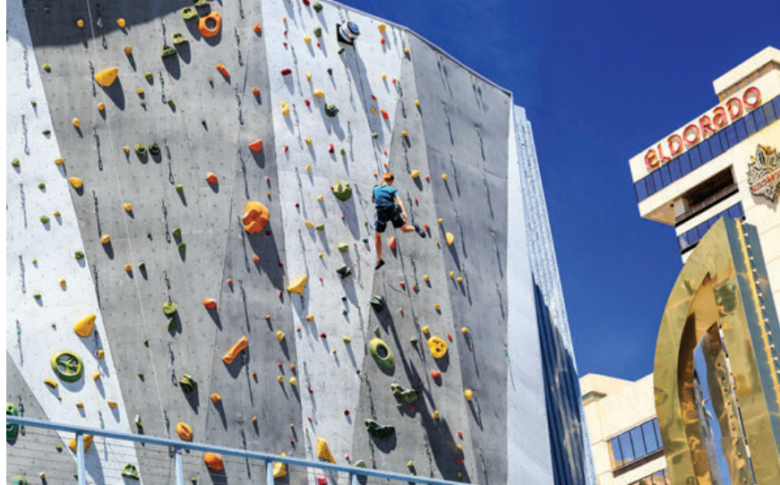
Climb up and ride down on BaseCamp Reno's outdoor climbing wall at Whitney Peak Hotel. The 164-foot-tall outdoor structure affords a great view of the area from the top.
