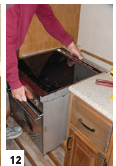
[9] Always measure twice before cutting. [10 and 11] Predrill all of the woodwork before reinstalling the mounting screws. [12] Proper installation of the new SMEV required a bit of patient manipulation, as the new configuration of space was rather snug.
