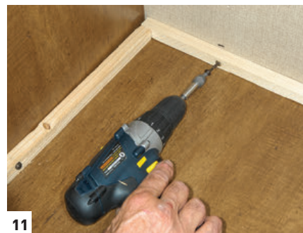
[9] Always measure twice before cutting. [10 and 11] Predrill all of the woodwork before reinstalling the mounting screws. [12] Proper installation of the new SMEV required a bit of patient manipulation, as the new configuration of space was rather snug.
