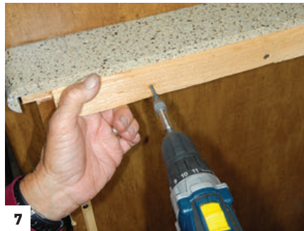
[5] Rubber gas lines are susceptible to damage caused from protruding staples and screws, so be sure to keep them out of harm's way. [6] When working with wood, exercise patience. Cabinet modifications will need to be made, and there is not much room for error. [7] The SMEV is roughly 1½ inches narrower than the original range, thus requiring a spacer board to be installed on both sides of the cabinet to fill the gaps. [8] Both spacer boards required sanding for a precise fit.
