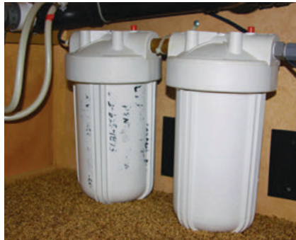
These two jumbo canisters contain a .5-micron ceramic filter and solid-carbon-block filter. Used in conjunction with one another, this is one of the best filtration methods on the market today.
