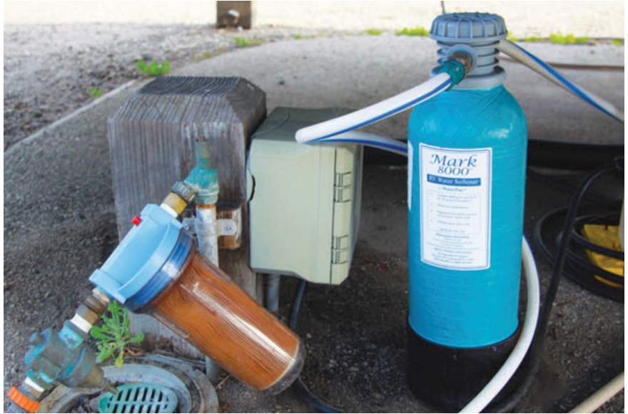
From left to right is a residential-style water-pressure regulator, a sediment and rust filter, which is easily cleaned and reused, and an RV-style water softener that keeps interior appliances and the shower spot-free.
