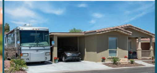
RV STORAGE PADS
