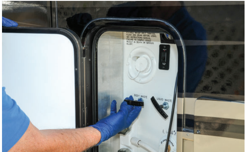
Keep valves closed except to dump. When dumping, open the black valve first and flush the tank, then close that valve and dump the gray tank, which flushes solids out of the sewer hose.
