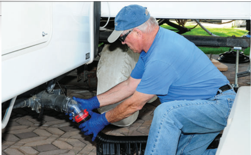
It's best to have a clear 45-degree elbow connector at the termination valve to see what is coming out of the tank, and to ensure the tank is clean. Use gloves and eye protection when flushing tanks.
