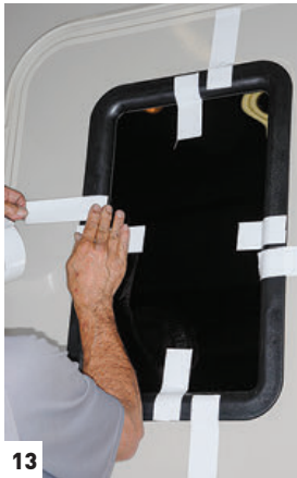
[13] Use duct tape to hold the glass and outer frame in place for a one-person job. [14 and 15] Install the inside frame top side up and do not overtighten the screws. The plastic frame will certainly crack when overtightened.
