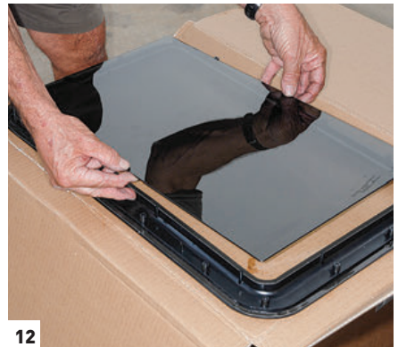
[7 and 8] Pull gently while removing the original inner and outer sealing tape to prevent leftover pieces. [9] Gently remove the original glass from the outside frame. [10 and 11] Install the new inner and outer seals, taking extra care not to damage the delicate material around the corners. [12] Set the new glass against the bottom stops and use your fingers to center the glass for a final installation.
