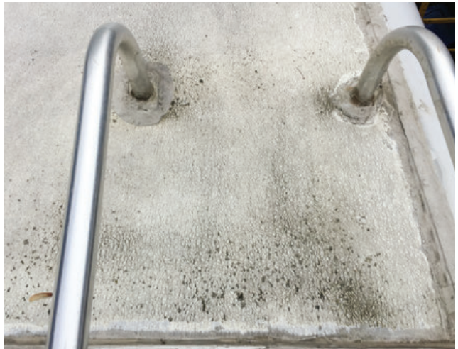
Above from left: Plumbing vents and skylights are common culprits for roof leakage and damage. Motorhome roof ladders are especially susceptible to seam cracking, since movement and stress when someone climbs the ladder impact the sealant.
