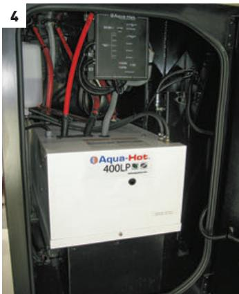
[4] The boiler tank is fitted in a prepared cabinet. The control panel is mounted above the main box. It provides all the diagnostic information. [5] Access to this heat exchanger is through the floor of a cabinet structure. [6] Nice-looking heat exchanger grilles are used to blend in with cabinetry.
