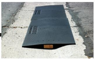
Above: Once the planks are attached, the mats are configured to fill in the gap in a rolled curb. The mats are fairly heavy, so moving them is not practical, nor is it necessary.
