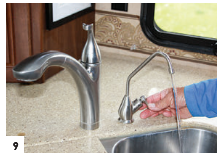
[7] Carbon filters used in the jumbo canister last much longer and will not restrict water flow. [8] In-line filters will help, but are designed for light-duty use in motorhomes that are used infrequently. Always look for an in-line filter with KDF additives, which help retard bacterial growth. [9] Filters that purify water can be routed through an independent faucet that's used for drinking and cooking. In most cases, it's not necessary to purify water for the entire motorhome, which will shorten the life of a carbon and/or ceramic filter.
