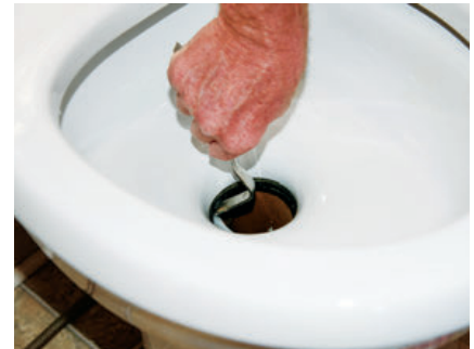
Use a coat hanger or other thin metal object with a smooth end to clean the inside groove of the toilet valve seal.
