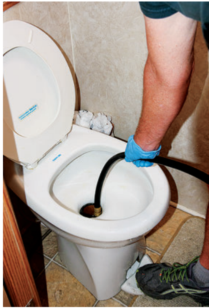
To ensure that all solids below the toilet are dislodged, direct fast-running water into the black tank via the toilet.
