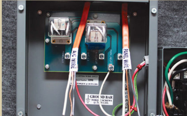
This smaller box houses the 20-amp breaker for the 30-foot power cord. Make sure the cord is securely clamped in place.
