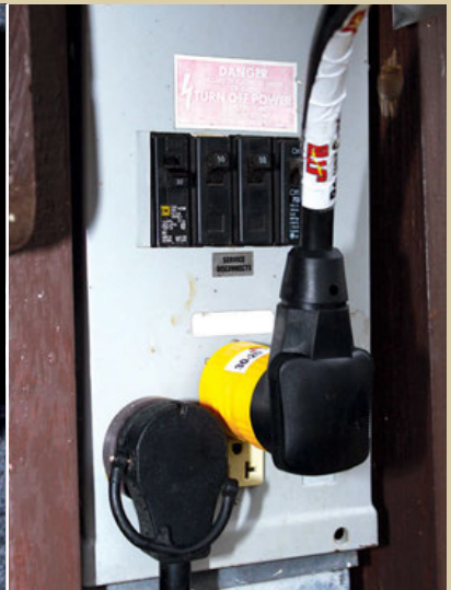
The JTB power cord with adapter is plugged into the GFCI, alongside the 30-amp power cord from the RV.
