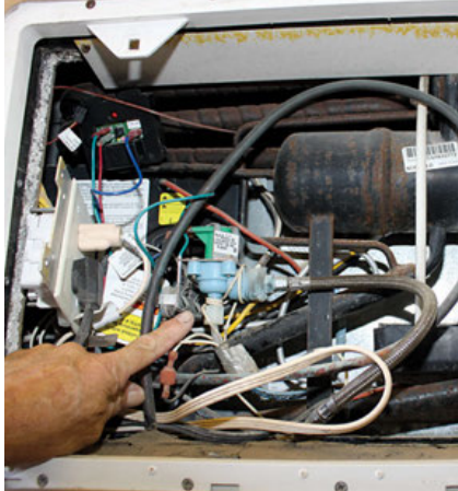
The water valve for the icemaker sits in a harsh environment and is often overlooked during inspection. Plastic lines on the inlet and outlet are susceptible to becoming brittle from heat and cold.
