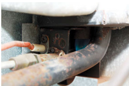
After servicing the refrigerator, you should see a blue flame without any trace of yellow.
