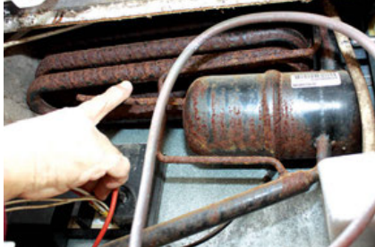
Excess rust will likely cause an early failure of this cooling unit.
