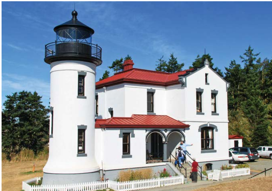
The decommissioned Admiralty Head Lighthouse at Fort Casey State Park was built with 18-inch-thick walls to withstand the concussions from the fort's big guns.
