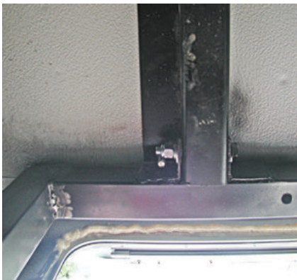
Two angle brackets were welded to the battery tray frame to provide an attachment to the body support that extends from the motorhome chassis.
