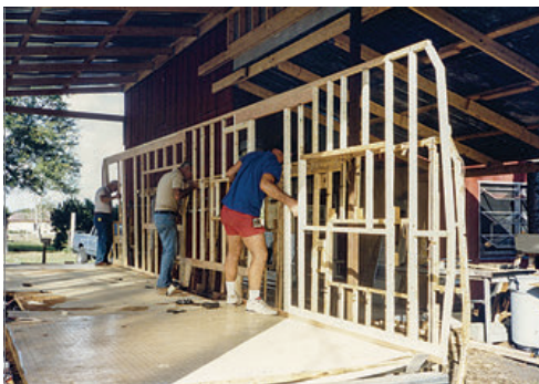
(Above from left) More than two decades ago, family and friends helped raise new walls on the floor of a wrecked trailer. Today, the trailer's interior looks as good as new.
