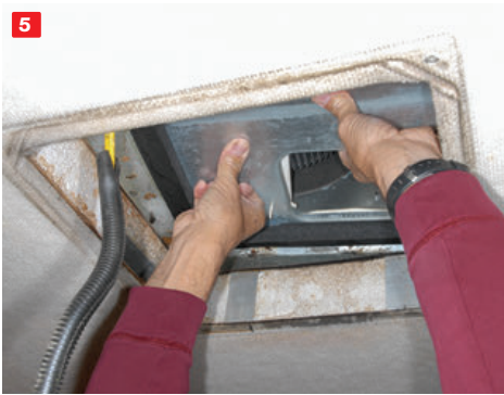
(4) The tie-down bolts holding the air conditioner in place can be quite long, so we opted to use a cordless drill for removal. (5) Apply steady upward pressure to break the air-conditioner gasket loose from the roof material. (6) This particular roof sagged a little bit and water had pooled under the air-conditioning unit. Be sure to remove any excess water before continuing on with the repair.
