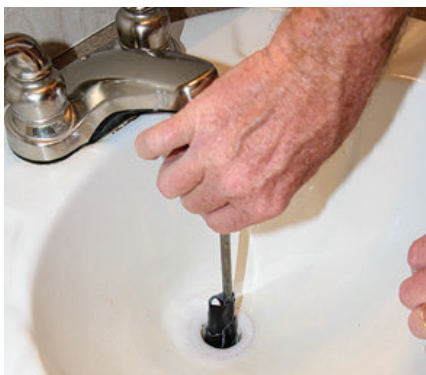
(Above from left) An old toothbrush is a great tool for scrubbing the vanity sink stopper. Tape an old toothbrush to a long stick (we use a tent stake) to scrub deep down inside the vanity sink drain.
