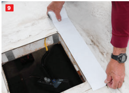
(7) As you can see from the lifted rubber, the faulty old gasket was causing a water leak. (8) Use Mineral Spirits to clean the gasket area when household cleaners won't do the job. (9) Rubber roof material can easily become damaged while extracting the air conditioner. EternaBond tape can be used to make the repairs. This will make a permanent seal. (10) A heavy-duty putty knife with a sharp edge is used to remove the old gasket.
