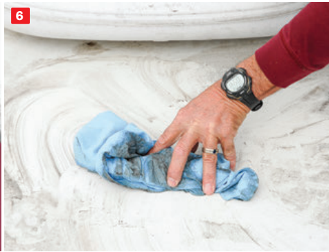
(4) The tie-down bolts holding the air conditioner in place can be quite long, so we opted to use a cordless drill for removal. (5) Apply steady upward pressure to break the air-conditioner gasket loose from the roof material. (6) This particular roof sagged a little bit and water had pooled under the air-conditioning unit. Be sure to remove any excess water before continuing on with the repair.
