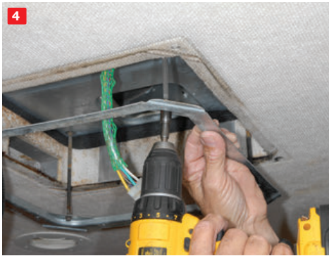
(4) The tie-down bolts holding the air conditioner in place can be quite long, so we opted to use a cordless drill for removal. (5) Apply steady upward pressure to break the air-conditioner gasket loose from the roof material. (6) This particular roof sagged a little bit and water had pooled under the air-conditioning unit. Be sure to remove any excess water before continuing on with the repair.
