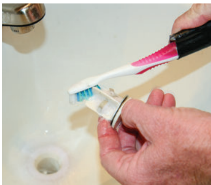
(Above from left) An old toothbrush is a great tool for scrubbing the vanity sink stopper. Tape an old toothbrush to a long stick (we use a tent stake) to scrub deep down inside the vanity sink drain.
