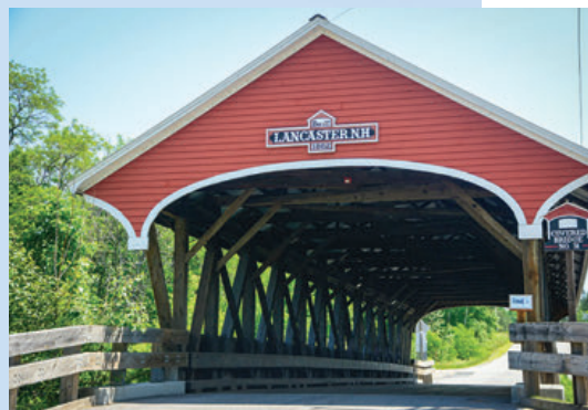
(Top and above) Built in 1862, the beautiful Mechanic Street Bridge in Lancaster is also known as the Israel River Bridge. It connected the mechanics of the town with the farmers across the river.
