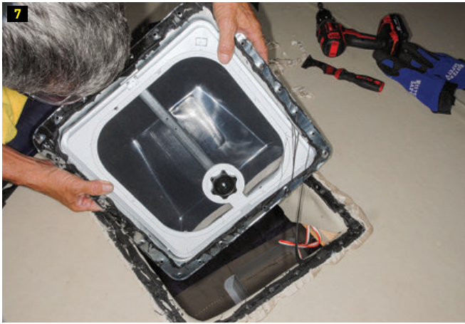
(7) The original roof vent is lifted off the roof. In this case the sealant was pretty fresh, so it was messy to work with. (8) A scraping tool is used to remove excess sealant from the rubber membrane surrounding the hole in the roof. Go slowly and use caution to prevent cutting the membrane.
