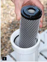
5) A sediment filter is used in the canister closest to the water source. Compare the filter in the canister to the new filter on the left; after only five weeks of service, it's easy to see why a sediment filter is needed. The filter should be replaced when water flow slows down. 6) A charcoal filter is used in the second canister. This filter will remove lead, heavy metals and cysts that taint the water and contribute to bad taste.
