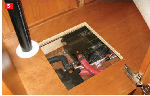
(4) Boiler tank is fitted in a prepared cabinet. Control panel is mounted above the main box. It provides all the diagnostic information for smoothing operation. (5) Access to this heat exchanger is through the floor of a cabinet structure. (6) Nice-looking heat exchanger grilles are used to blend in with cabinetry.
