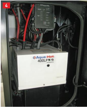
(4) Boiler tank is fitted in a prepared cabinet. Control panel is mounted above the main box. It provides all the diagnostic information for smoothing operation. (5) Access to this heat exchanger is through the floor of a cabinet structure. (6) Nice-looking heat exchanger grilles are used to blend in with cabinetry.
