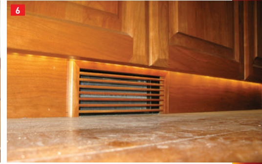
(4) Boiler tank is fitted in a prepared cabinet. Control panel is mounted above the main box. It provides all the diagnostic information for smoothing operation. (5) Access to this heat exchanger is through the floor of a cabinet structure. (6) Nice-looking heat exchanger grilles are used to blend in with cabinetry.
