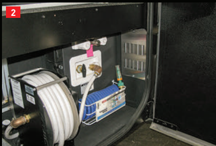
(1) Rather than using standard issue heat ducting, the Aqua-Hot relies on a network of 5/8-inch PEX tubing that's routed to individual heat exchangers. (2) Typically, a heat exchanger is installed inside the utility bay. (3) Here the backside of the heat exchanger can be serviced from inside a neighboring compartment.
