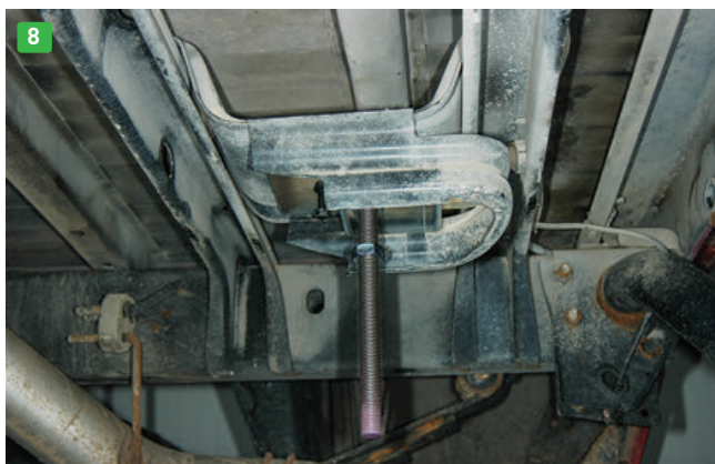
(8) The truck-mounting plate is bolted to the old spare-tire winch location using supplied fasteners. (9) The Titan tank is prepped on the bench by adding the hose fittings; location is obvious, and the fittings are simply angled in the direction necessary for best hose routing.
