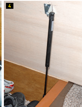
3) The bottom bracket is installed using wood screws. Here, there was plenty of wood backing to facilitate a strong connection. 4) Gas struts are snapped on the ball ends of the upper and lower brackets.
