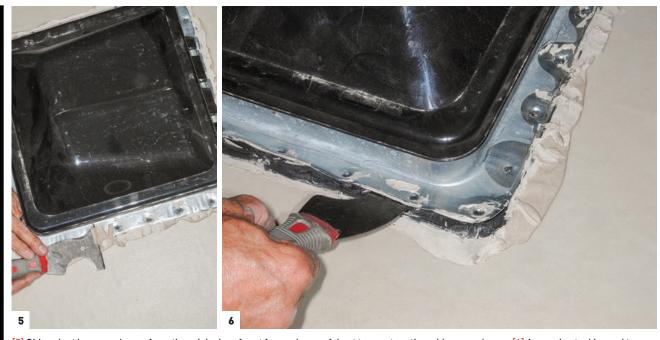
[5] Old sealant is scraped away from the original roof vent frame; be careful not to puncture the rubber membrane. [6] A scraping tool is used to release the factory roof vent from the roof. Take time to do it right and prevent damage to the rubber roof, which will likely lift up during the process.
