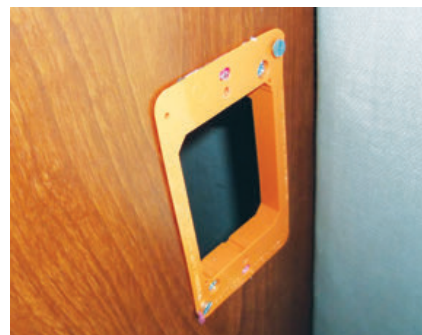
3. A backless box makes connections easier.
