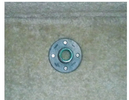
13. Locate and pilot drill for the floor-flange mounting screws.
