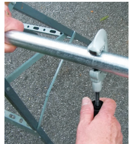
12. A tubing cutter makes a clean, straight cut on the 1-inch EMT conduit.
