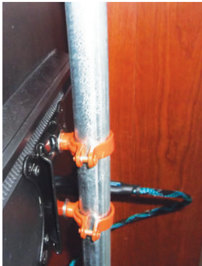
14. The split-ring hangers will hold the monitor and keyboard tray to the pole at any height.
