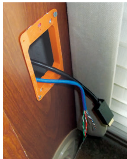
4. The paired wires of the CAT 6 cable will connect the speaker and microphone to the computer.
