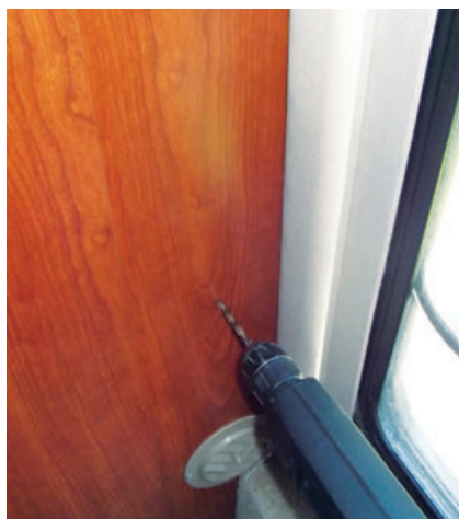
2. Pencil in the outline of the box and drill the corners to cut out with a keyhole saw.
